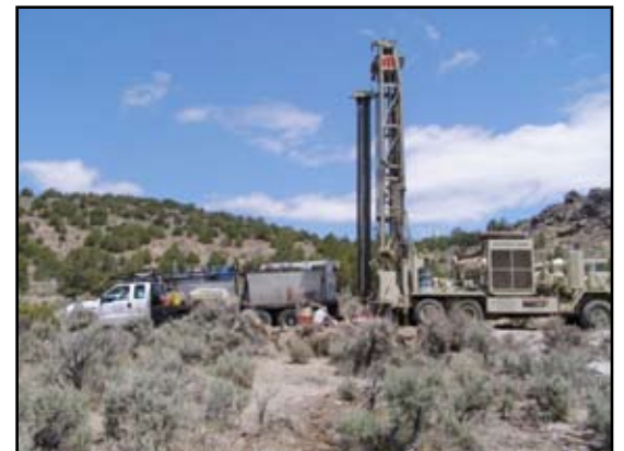
Bruce McKay was hired to dig a well on Ranch property. We hit water at 80 feet, revealing an actual oasis in the desert.
